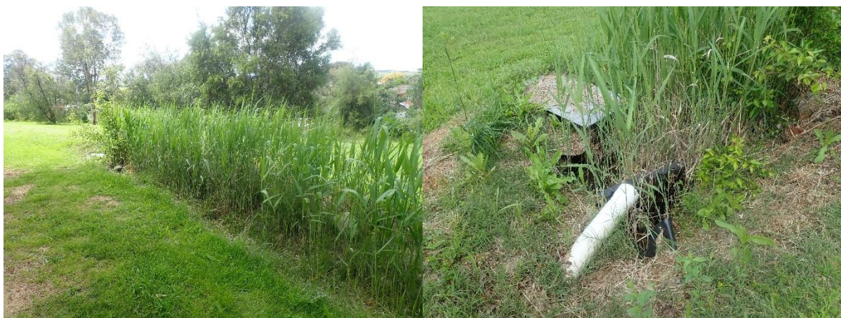
Figure 30 (left) greywater is treated in a Cumbungi wetland; (right) the pipe infrastructure needs maintenance if it is to function properly
